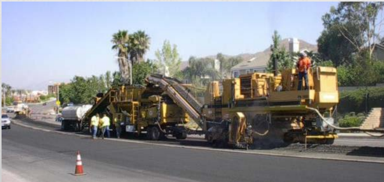
Cold In-place (CIR)
